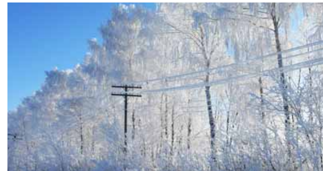
The ideal site for the reserve power plant is at the intersection of most of the country's main voltage lines in the small borough of Kiisa.
