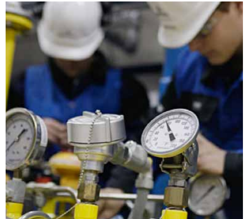
The new plant will become the African continent's largest to be based exclusively on gas-fired combustion engines.
