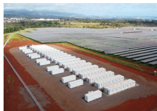
Clearway solar and storage power plant in Miliani, Hawaii.
